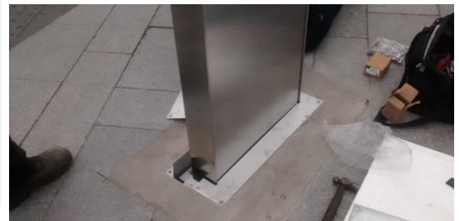
Base-box open with Monolith being installed with the two piece lid
