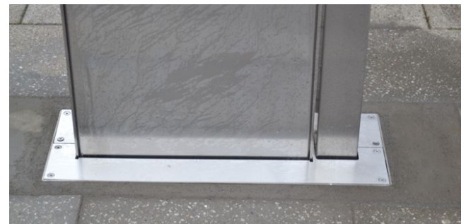
Monolith installed to Base-box with the 2 piece lid housing the monolith
