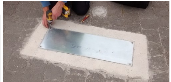
Base-box idle waiting for monolith to be installed
