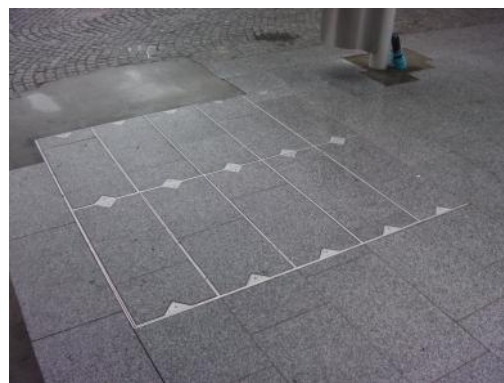
Grade 304 Stainless Steel Kent Telecover Paver installed in Sheldon Square, London (UK)
