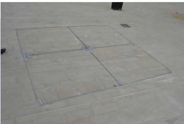
Grade 316 Stainless Steel Kent Hinged Multi-paver installed in Lusail City (Qatar)
