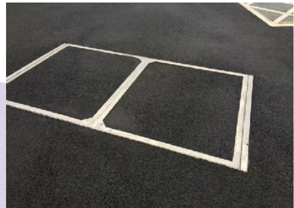
Grade 304 Stainless Steel Kent Multi-Paver installed in St. Barts Hospital, London (England)
