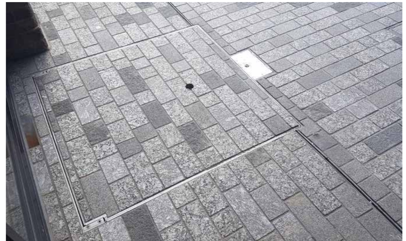
This Event Box is for major large scale events - such as plugging in an Ice Rink in addition to the regular food cart and lighting demand that accompanies this.
