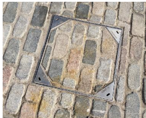
Grade 304 Stainless Steel Kent Solo Paver installed in Hemel Hempstead, London
