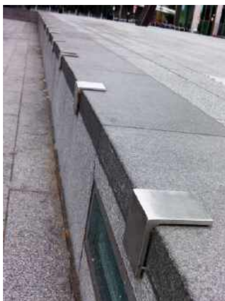
Angle Anti Skate Studs installed in Canada Water, London
