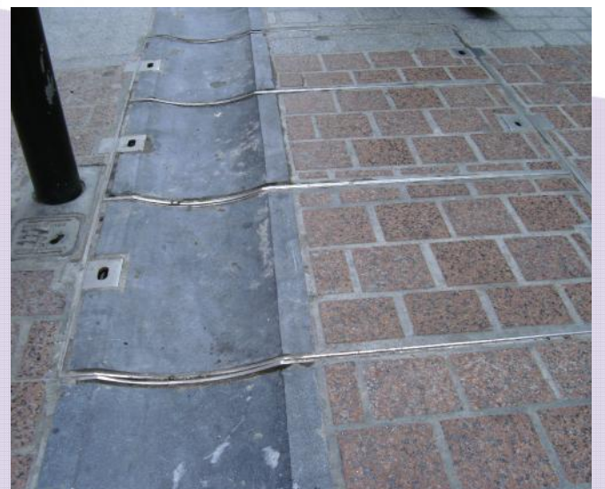
Dished Telecover installed in Main St, Wexford (Ireland)
