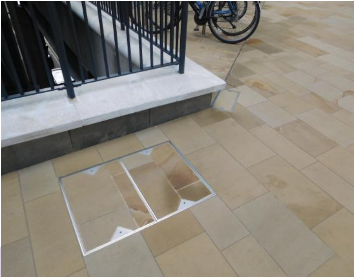
Muti Paver Telecover option installed in Letchworth
