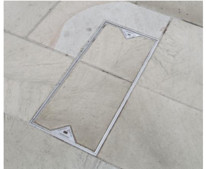
Single Paver Telecover option installed in Letchworth
