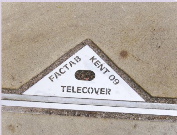
Laser cut lettering on Telecover lift-out point
