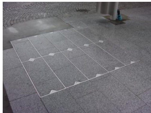
Grade 304 Stainless Steel Kent Telecover Paver installed in Sheldon Square, London (UK)
