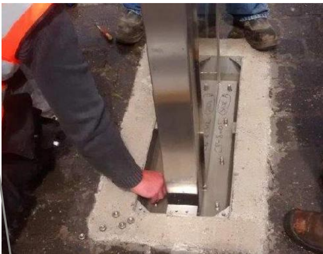
STAINLESS STEEL ACCESS COVER AND FRAME FOR MOUNTING ON SLOPING GROUND
