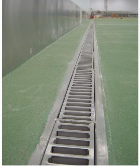
BS EN1253 Loading Class L15 / R50 / M125 / N250 / P400 Our <u>internal</u> factory gratings can be subjected to very heavy loads and the grating depth and bar thickness will be determined by Kent to suit your project. Suitable for Factories—Meat /
