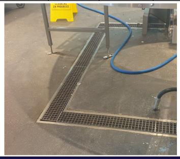
Specify: Kent Anti-slip Mesh Grating KAMG<u>150</u>; <u>150mm</u> wide grating; <u>990mm</u> long; Grade <u>304</u> Stainless Steel; Load Class <u>B</u>
