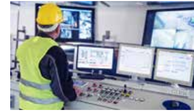
Activated by Control Room
