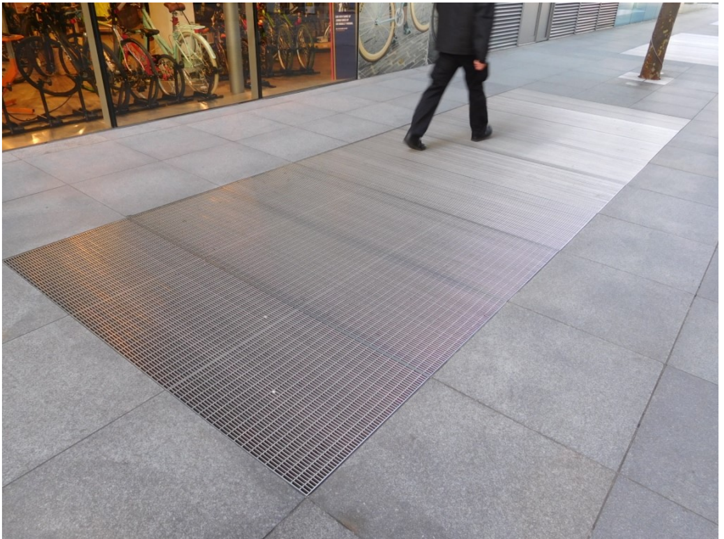
Regent's Place, London—5mm Bar / 8mm Gap. 6m long x 2250mm wide. FACTA B Loading
