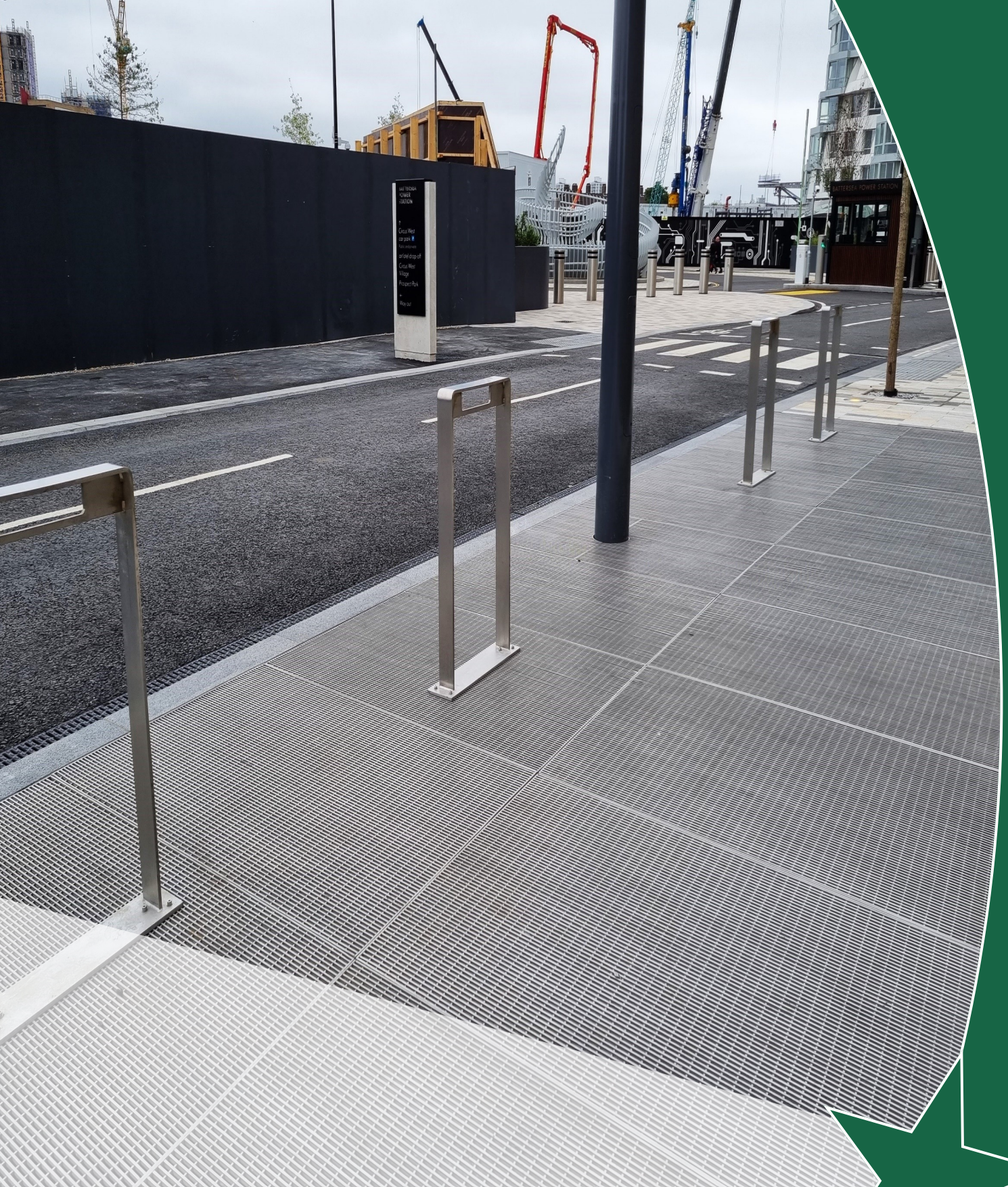
Sea Power Station, London—5mm Bar / 8mm Gap. 12m long x 2.2m wide. FACTA B Loading (also showing Stainless Cycle Stands)
