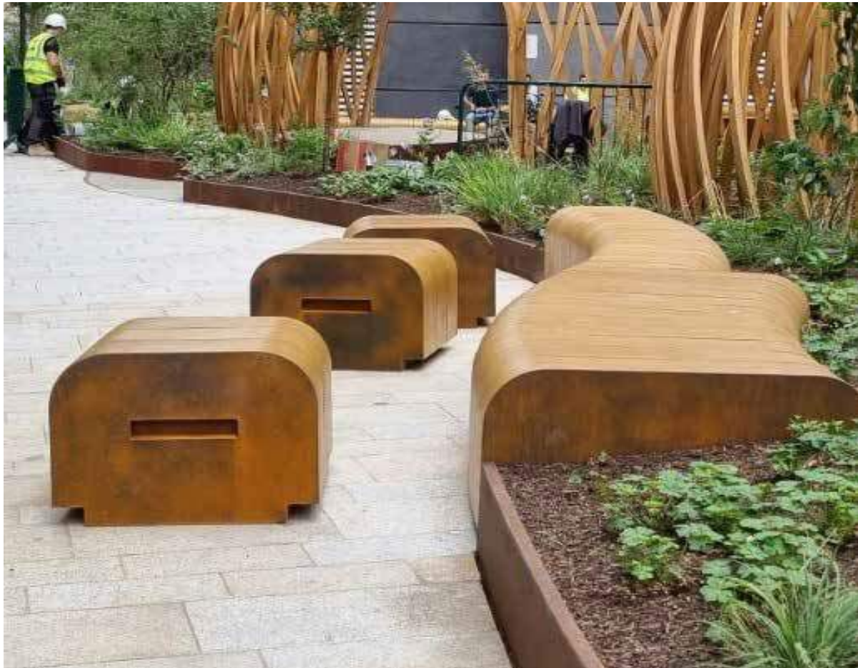
Glue Laminated Timber Seats with Pre Weathered Corten Side Panels—Triton Square, London UK
