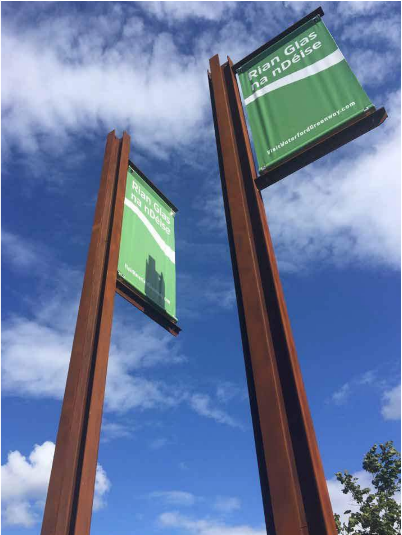
Waterford Greenway Banner Poles—Waterford (structural steel)—Corten B
