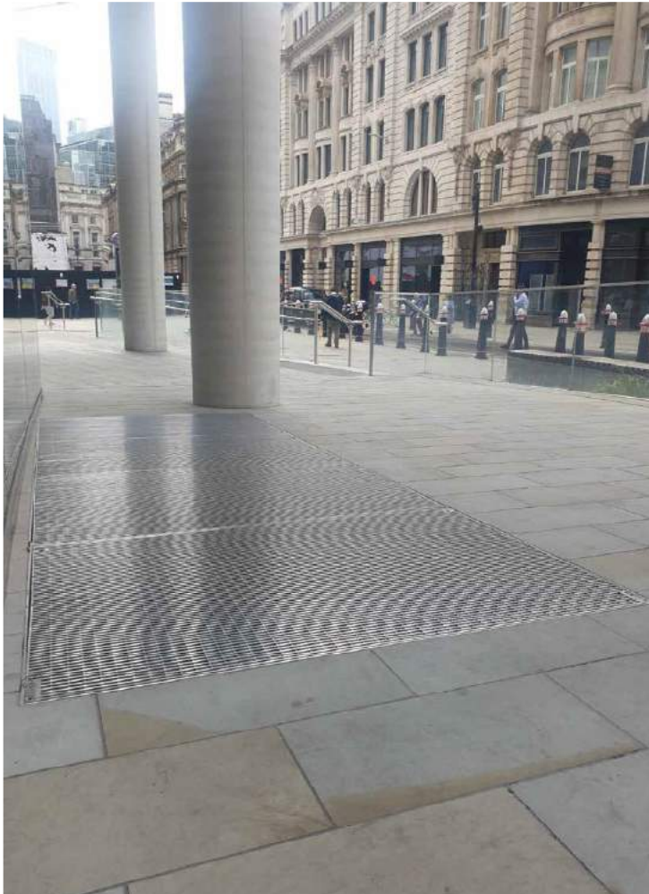
Heelproof Ventilation Grilles—100 Liverpool St, London
