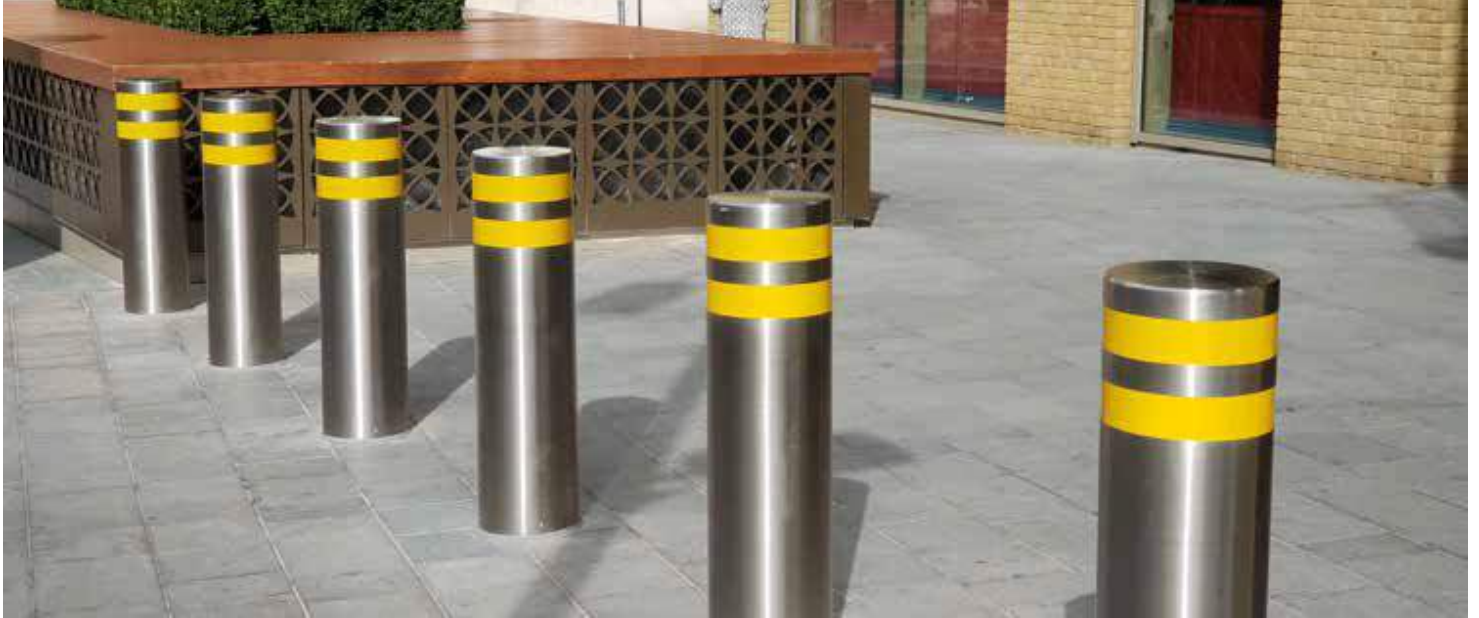
PAS68 Bollards—One Tower Bridge, London
