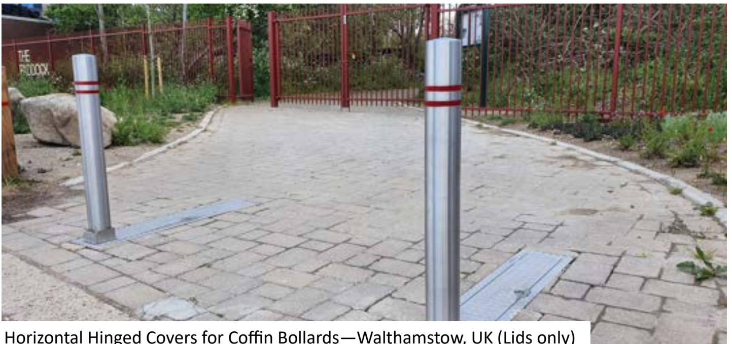
Vertical Ventilation Panels between steps - Battersea, London
