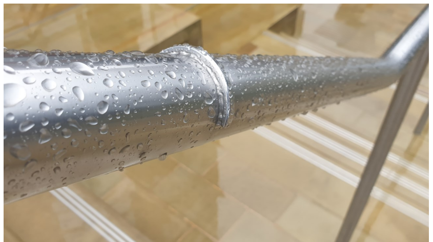
Anti-skate rail welded onto handrail
